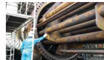
PREST/ON-SITE SERVICES We offer a complete range of on-site solutions, including flange integrity management, technical assistance, and on-site machining.
