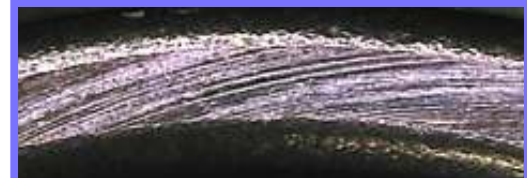
POOR FLANGE FINISH - RADIAL MARKS
